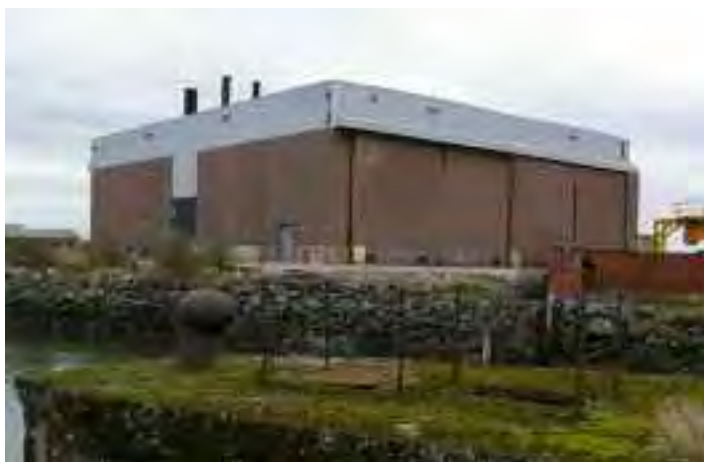
Paint Hall in Belfast's Titanic Quarter
